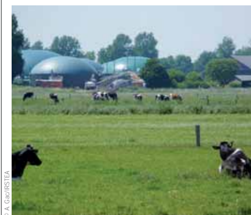
A methanation plant in Germany.
