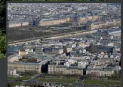
Research measures the impact of climate change on various urban developments, providing precious data for urban planners. © Pascal Taburet/Météo-France
