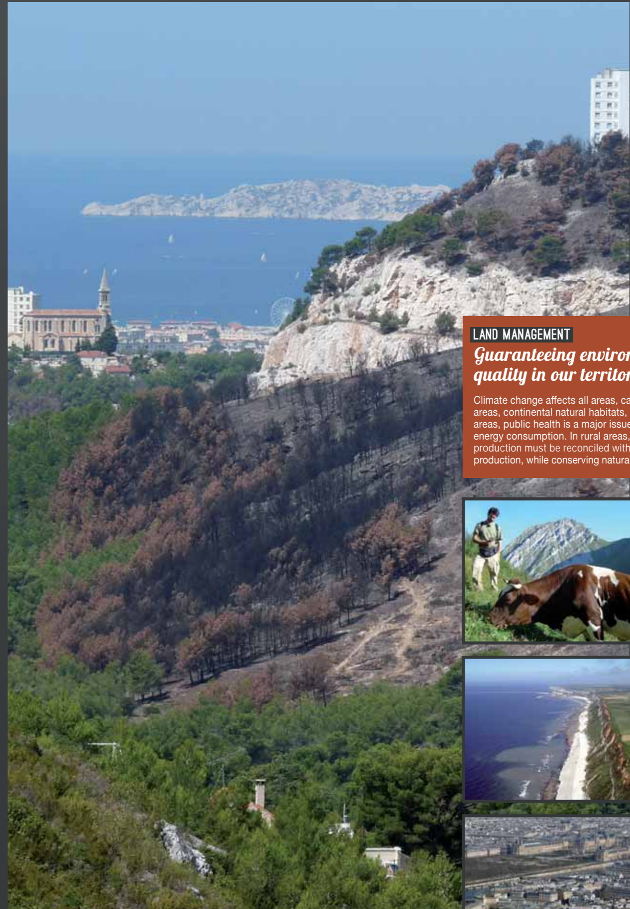
Damage observed in the built environment in Marseille following the wildfire on 22 and 23 July 2009. © Marlène Long/IRSTEA
